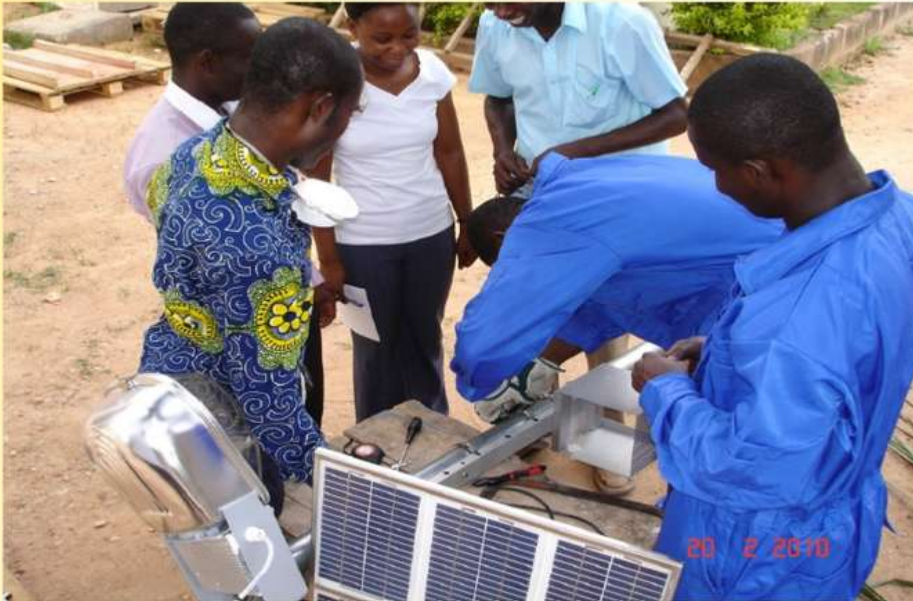
Solar Street light installation training
